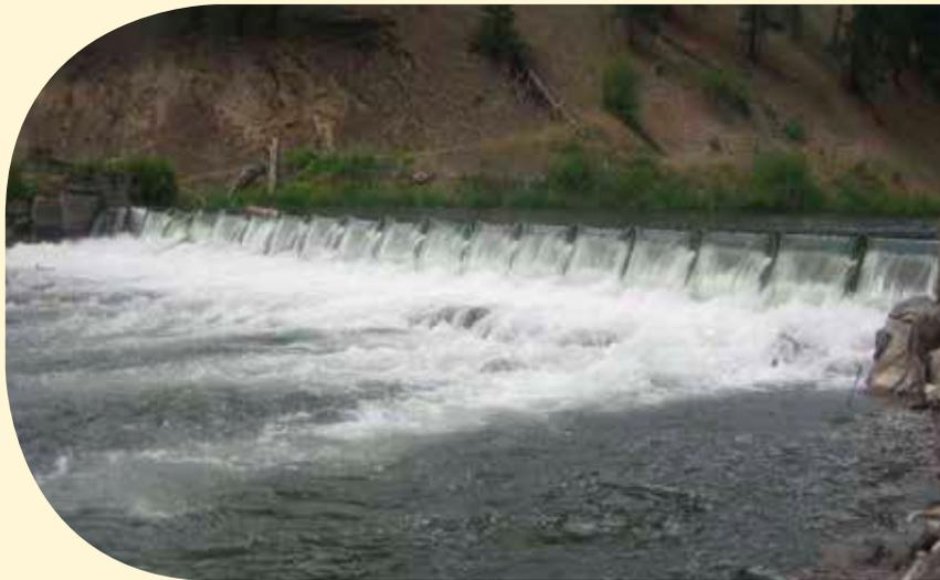
French-Grass Valley Diversion Dam on the Clark Fork just west of Missoula - diversion dams can be dangerous when flash boards are installed, creating a large drop and unpredictable conditions below.
